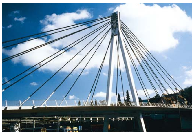
Figure 10 - Storchenbrücke in Winterthur
